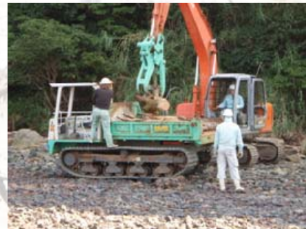
Cleaning by heavy machinery
