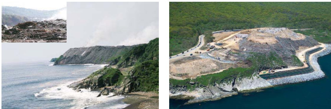
Figure 7. Gornostay Bay dumping site in 2009 (left) and the renovated dumping site in 2011 (right)
