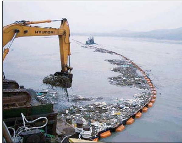
Figure 4. Removal of marine litter collected by a trash boom in Incheon City
