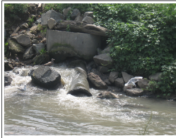
Fig.4.2 Inputs of untreated waste waters into Vtoraya Rechka which inflow into Amursky Bay.
